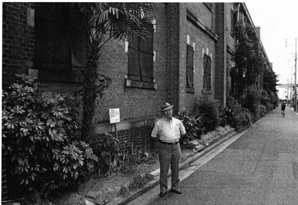
Hibakusha Keijiro Matsushima is shown in 2010 standing in front of the former Hiroshima Army Clothing Depot where he was forced to work during the summer of 1945 before becoming a student at the Hiroshima National Technical College. Although this structure is almost 1.75 miles from the Hypocenter, most of the heavy steel covers over the windows were blown inward by the massive shockwave. (Author)
