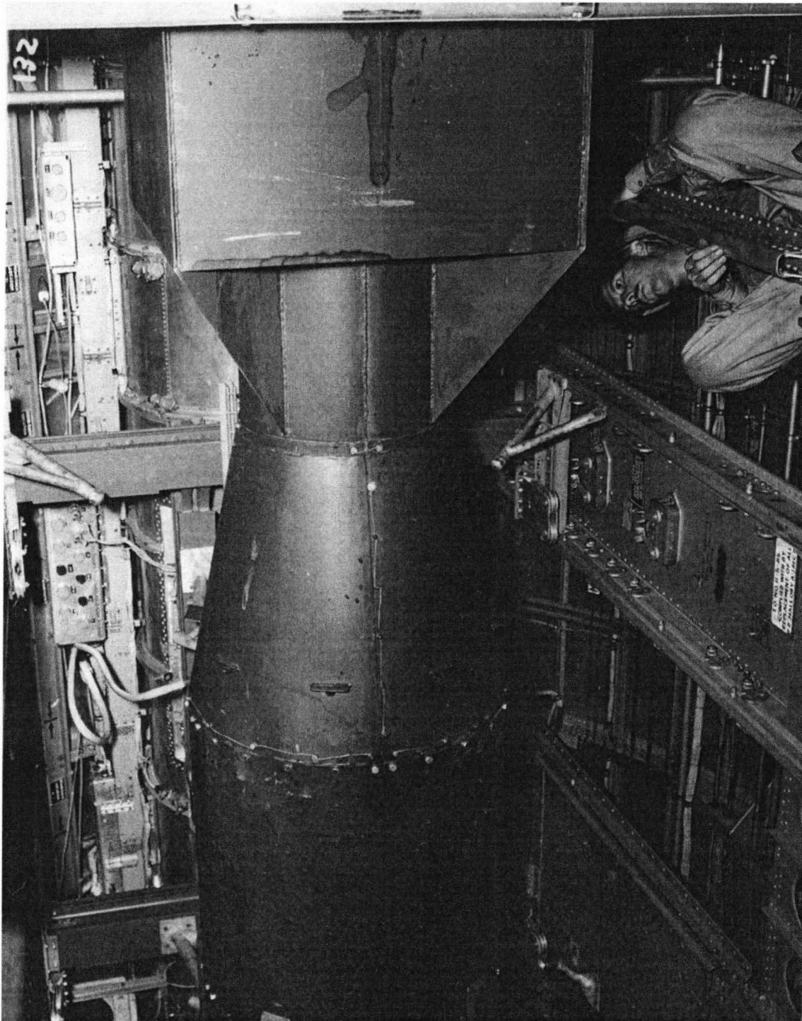
View looking up into Enola Gay after L-11 was loaded into the bomb bay. Sheldon Dike is visible on the right. Note the safety wires attached to all of the bolts on the tapered section of the tail. The bottom edge of the removable platform used by Parsons to arm the bomb is visible at the very top of the photo. (National Archives)
