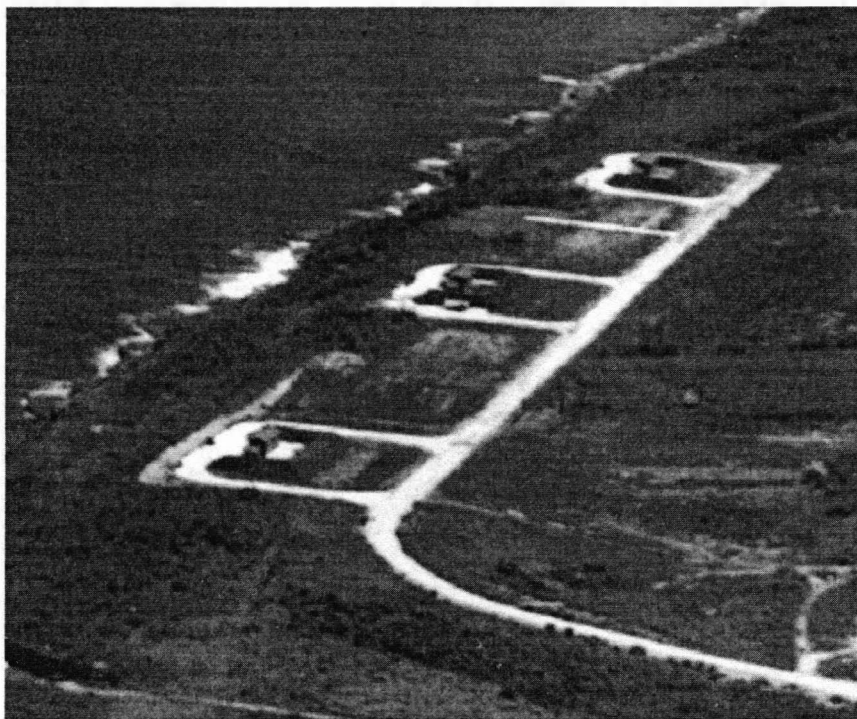
Here are the three bomb assembly buildings. The #1 building at the bottom is where Little Boy was assembled, #2 was used for assembly of the Fat Man test units, and building #3 shown at the top was used to assemble the F-31 combat Fat Man . The earthen berms are visible surrounding each building on three sides. (Leon Smith)
