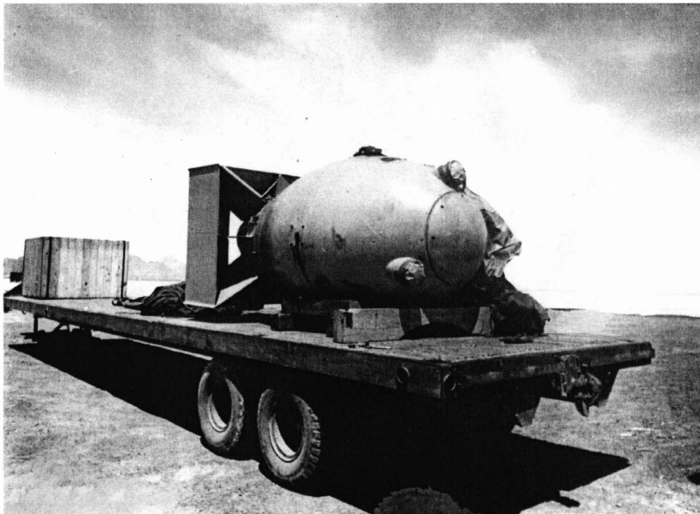
Pumpkin on trailer at Wendover. Note three nose contact fuzes instead of the four used on Fat Man . (LANL)
