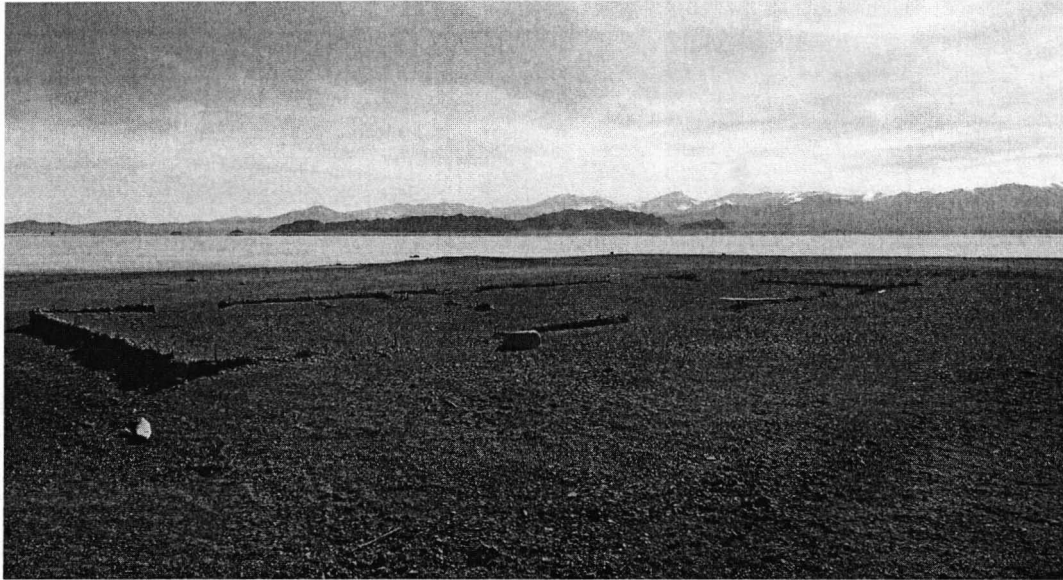
All that remains in 2005 of the Fat Man final assembly building are the footings and crumbling concrete floor on a cinder block pad spread over the Wendover desert. (Author)
