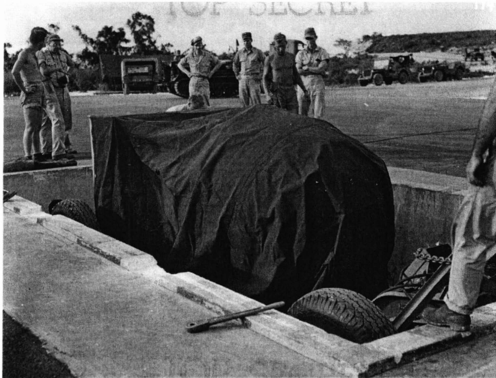
Canvas shrouded F-31 being lowered into pit. (National Archives)
