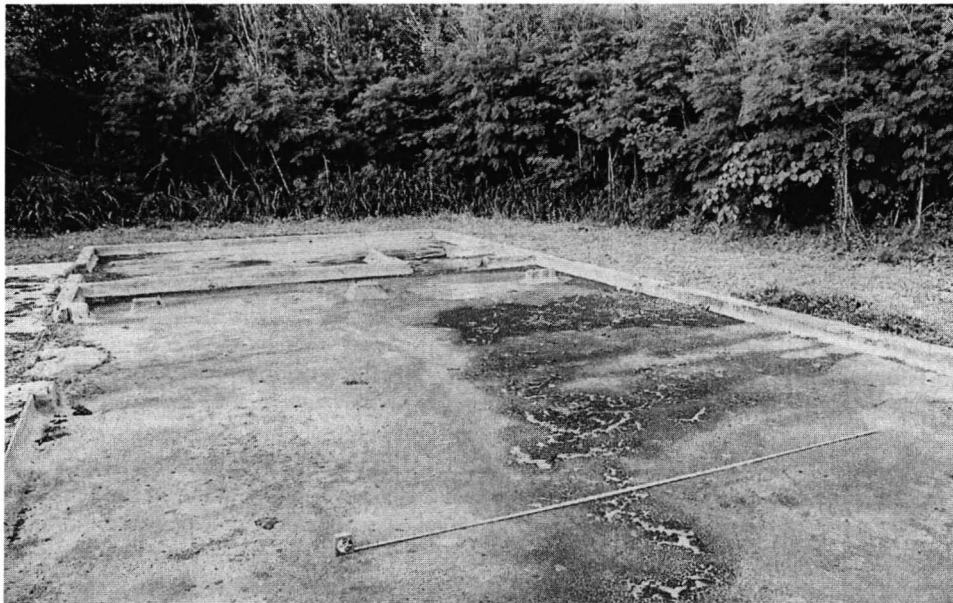
This is what the same Tinian assembly building looked like in August 2005. The structure itself was torn down by salvagers decades ago. What remains is the concrete floor and wall footings surrounded by dense jungle growth. The tape measure represents the placement of the LB unit in the 1945 photo. The area in the upper photo hidden behind the equipment cabinet is the double door leading to the outside concrete apron. The opening for that door is shown on the left side of this photo. (Author)
